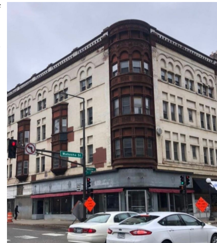
Exterior of building, before
