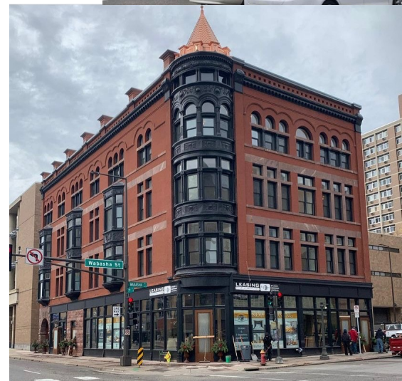
Exterior of building, after
