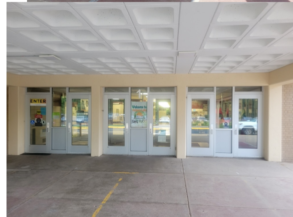
Top: Entrance prior to replacement Bottom: New replaced entrance
