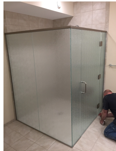
Right: One of the 24 shower enclosures after installation
